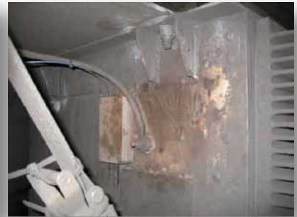
FBG Sensor on train rectifier
