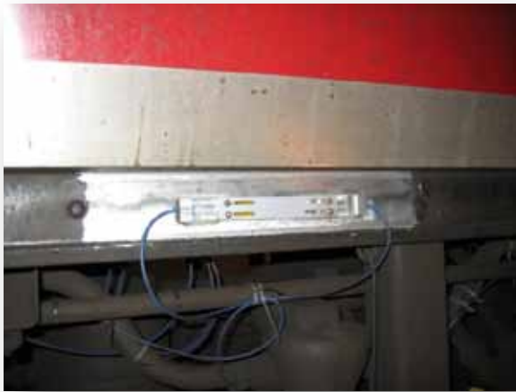
FBG Sensor on train solebar.
