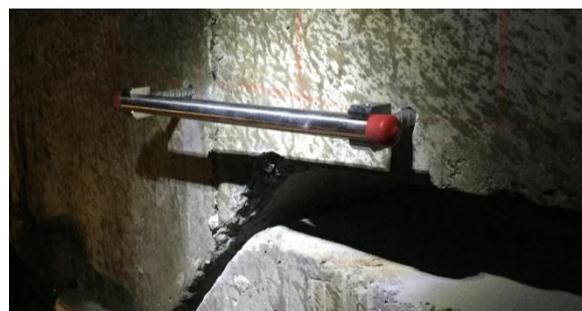
**Figure 4 Installation and Setting of the Sensor Anchors**
