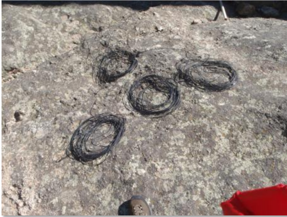
Installation of fiber cable runs for the four monitoring locations.
