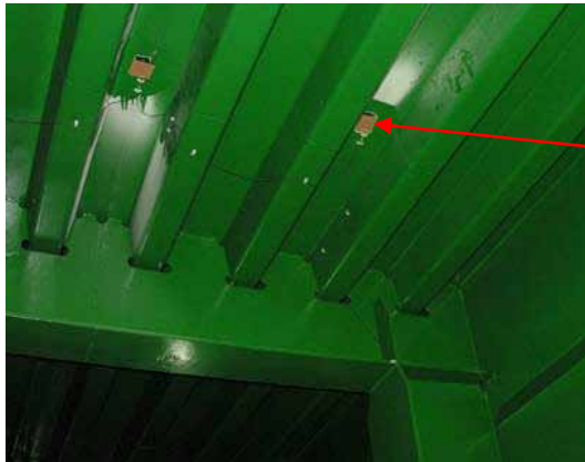
os3100 on truss ceiling..
