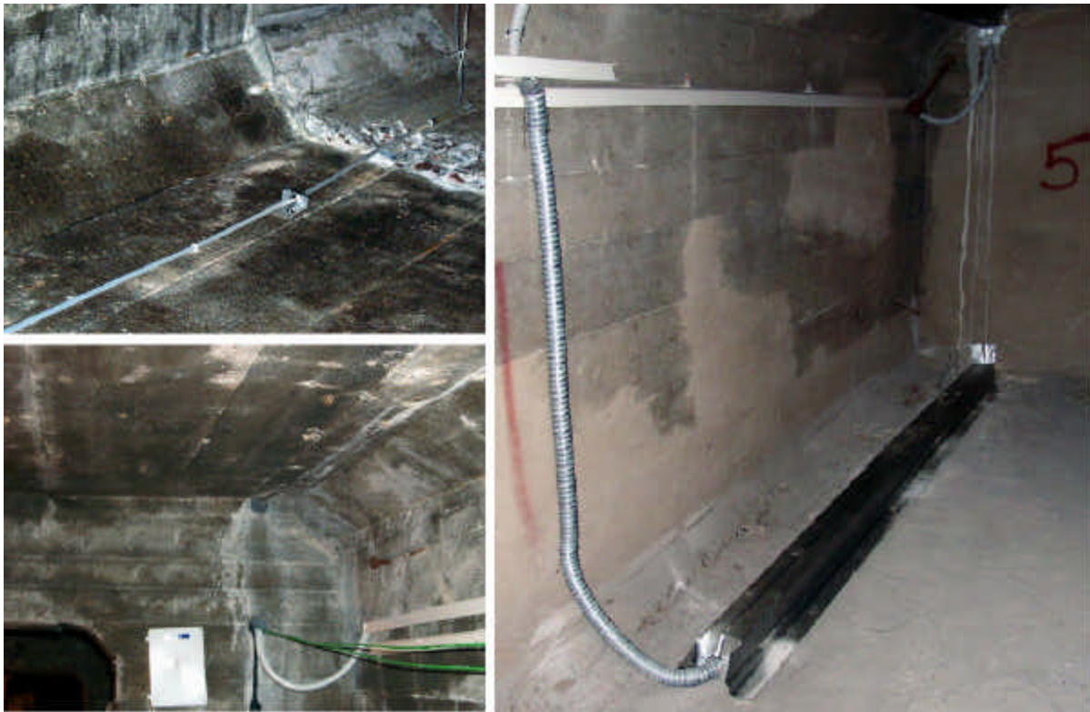
Figure 3. SOFO sensor before and after protective cover was installed.
