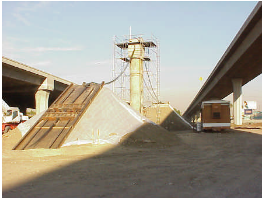
Figure 7. Bridge stack being prepared for destructive test
