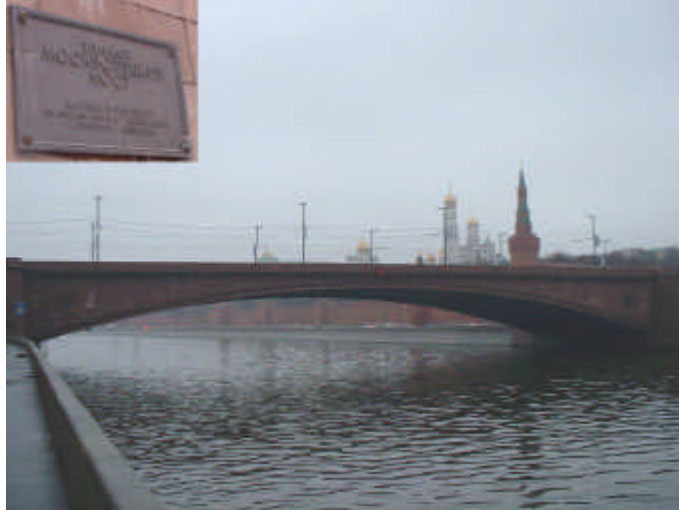
Figure 4. A full view of the Bolshoi Moskvoretskiy Bridge
