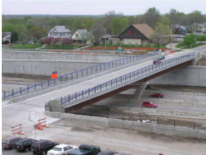
Figure 5. East 12 th Street Bridge as seen from SHM network camera
