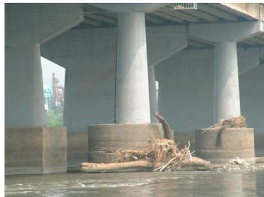
Figure 4 Debris trapped in front of the bridge piers
