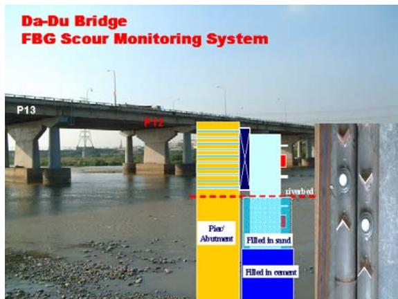
Figure 1 Installation of the FBG monitoring system in the Dadu Bridge
