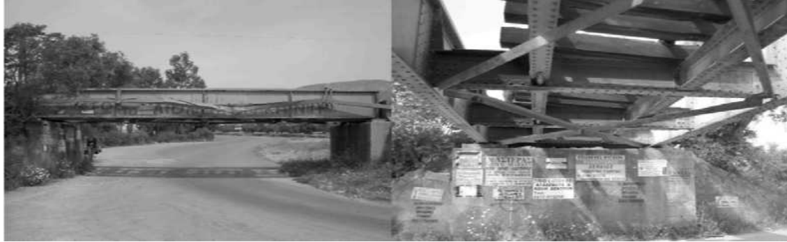
Figure 1 : Nea Peramos steel railway bridge
