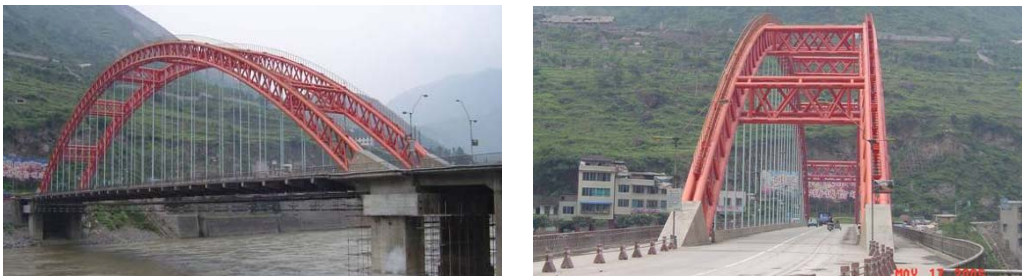
Fig.1. Ebian Daduhe bridge
