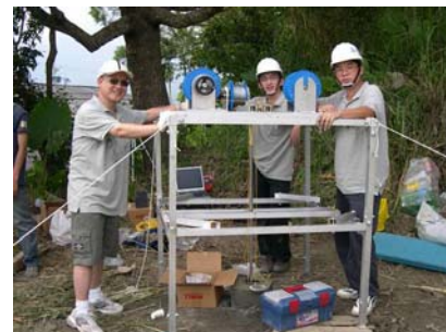
Fig. 3. FBG Bending Gauge installation work at the Chi-San Fault
