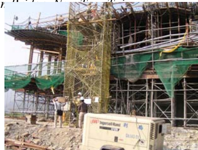
Fig. 7. Sensor installation at Ai-Lan Bridge
