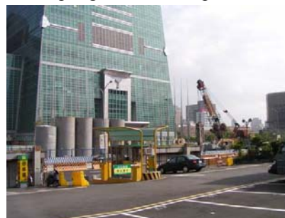
Fig. 8. FBG Bending Gauges to be installed at the MRT station site adjacent to Taipei 101
