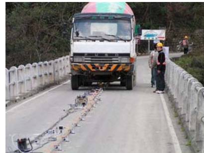
Fig. 1. Static loading test of the Hsin-Han Bridge
