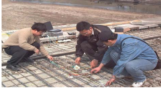
Fig.2. FBG sensor installation on bridge surface.
