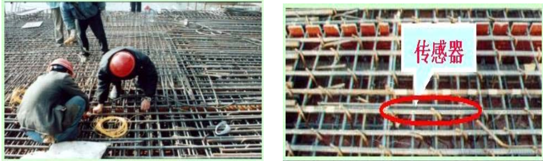
Figure 3 photographs of installing sensors
