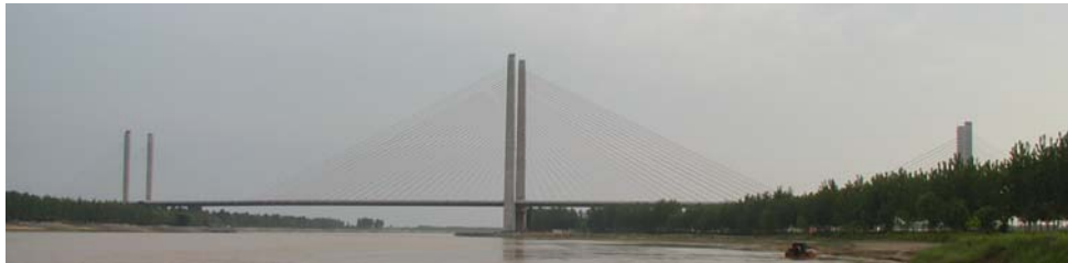
Figure 1 Binzhou Yellow River Highway Bridge
