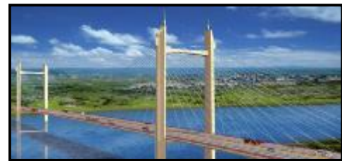
Figure 11. Songhuajiang River Bridge in Heilongjiang Province
