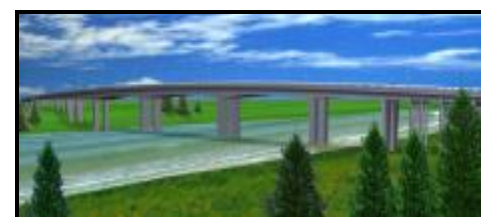
Figure 12. Dongying Yellow River Bridge in Shandong Province
