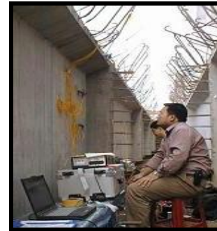
Figure 10. Niutoushan Bridge in Heilongjiang
