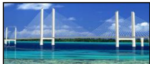
Figure 13. Binzhou Yellow River Bridge in Shandong Province
