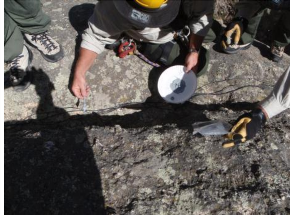
Securing the tie down clips to the rock with epoxy for securing the fiber cable runs.
