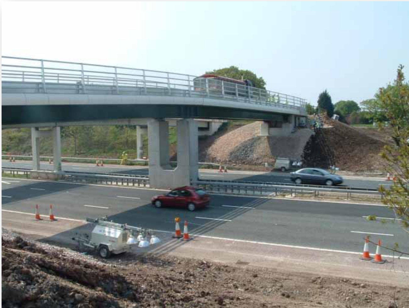
Composite motorway bridge
