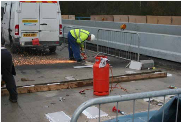
Installation of sensors on the bridge deck.
