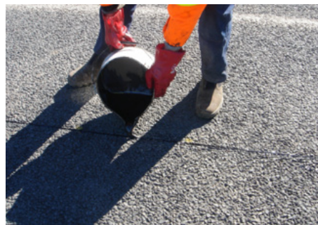
Epoxy resin poured around the 1 mm diameter cables in one application
