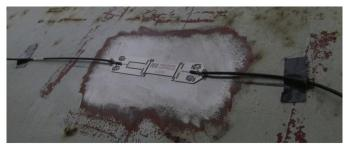
Luna's os3155 rugged fiber optic strain gages are installed along exterior steel pate girders to measure strains for loads that can run as high as 410,000 lbs.
