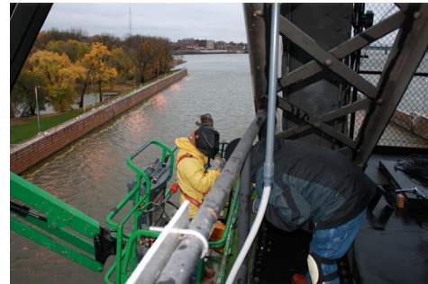
Access via man-lift and scaffolding
