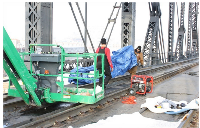
Sensors being prepped for installation
